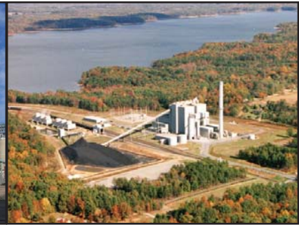
132 MW pulverized coal-fired plant in Virginia.
